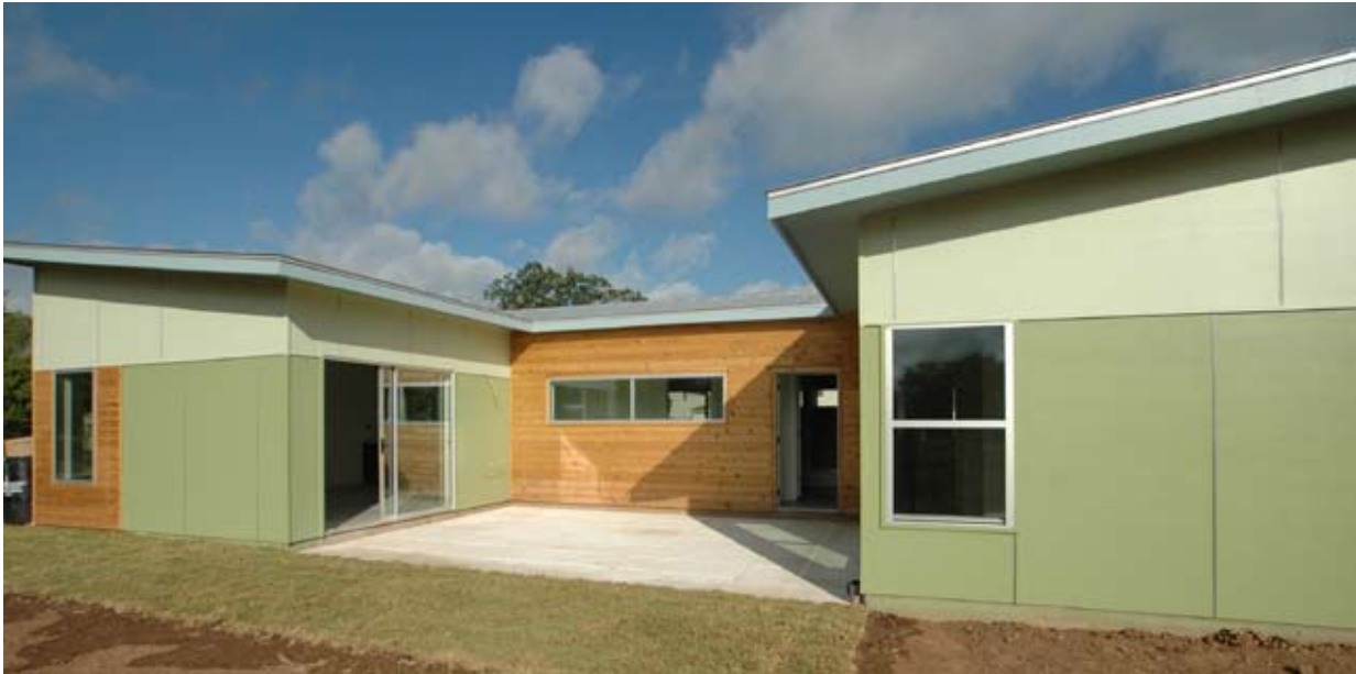
Architects KRDB are constructing a neighborhood made up of 38 net-zero energy homes on the eastern side of Austin. The neighborhood, entitled Sol Austin, or "Solutions Oriented Living," features homes designed to produce as much energy as they use in the course of a year through efficient construction and integrated solar energy systems. Photo: KRDB
