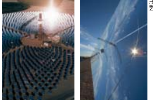
Solar Two (left), a power tower in the desert southwest, demonstrated the feasibility of storing heat from the sun to generate electricity at night. For over 10 years, parabolic solar trough power plants (right) have produced electricity for California.
